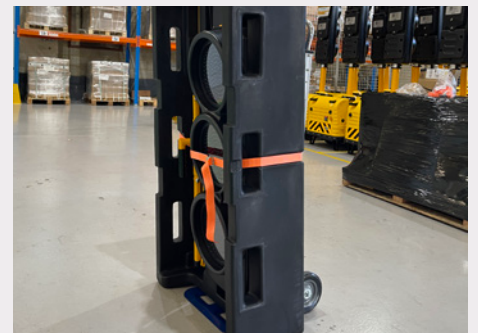
With the signal secure, move using a lightweight sack truck or carry the stillage flat with a second person.
