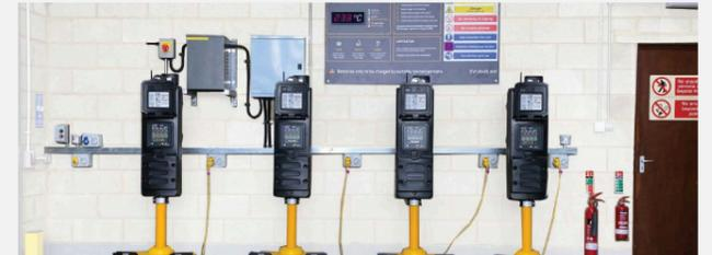
Explosive gases are given off when batteries are charged. The risk of an explosion is great if the gases are allowed to collect. When charging batteries, ensure you have a suitable Charging Station by following our guide.
