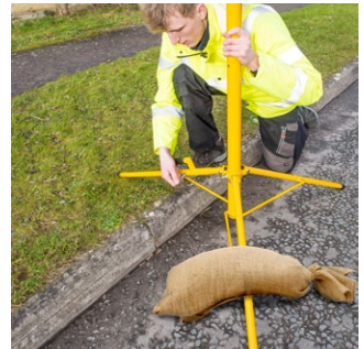
In high wind conditions use sand bags to secure the signal.
