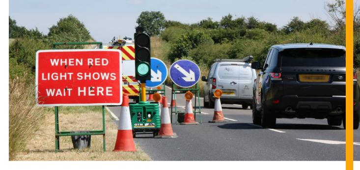
RadioConnect2's secret weapon is AutoGreen technology, which uses information from an advanced onboard radar sensor from AGD Systems to measure the amount of traffic queuing and automatically adjusts green times accordingly. It doesn't just protect staff though – it keeps motorists happy too. It's highly frustrating to be stuck on red at portable traffic lights when you can see there's nothing coming the other way.
